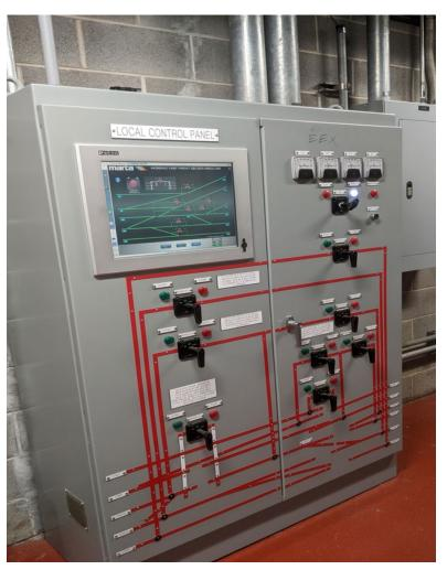
Local Control Panel (LCP) with HMI Screen
